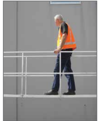
TREADPLANK WITH HANDRAIL
