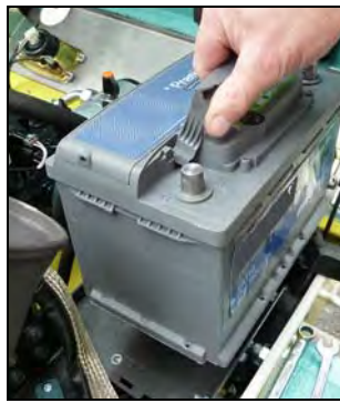
Fig. 10-2 Replacing the battery
